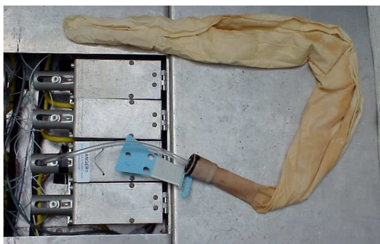
Figure 37. Completed balloon assembly with cable tie trimmed, ready for inflation.
