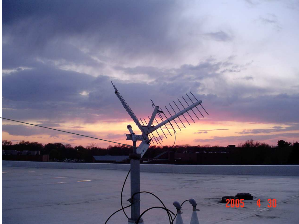
Figure 20. System 403 MHz RF telemetry down link antenna. The mast can be manually turned in the direction of the upper air winds to maximize long range downwind telemetry reception. Note weather head entrance for coax on roof.
