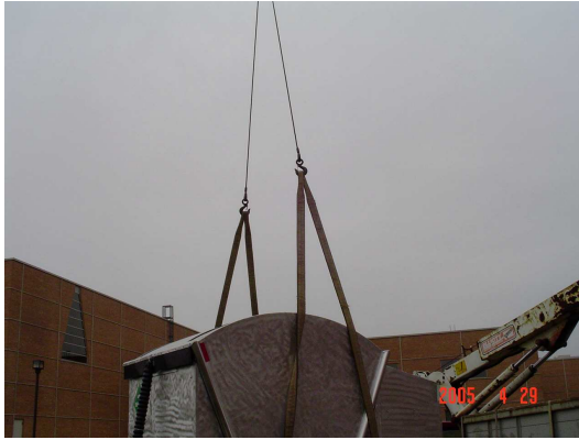
Figure 15. Crane lifting the ARL-9000 onto a roof.
